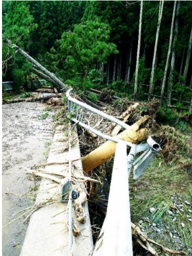
Yatabe Bridge over the Takatoki River. August 5.
